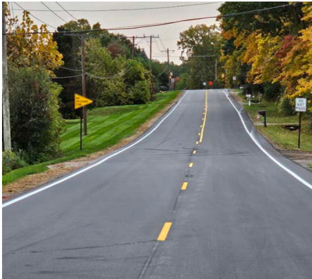
Textile Rd between Crane Rd & Munger Rd (Ypsilanti Twp), 2023
